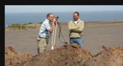
Grant Bland and Mark Muller check levels at their latest project.
